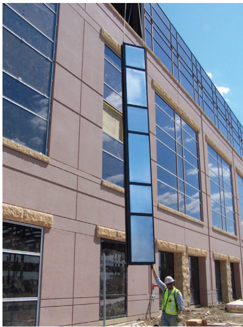
Unitized Panel Installation Wells Fargo Home Mortgage West Campus
